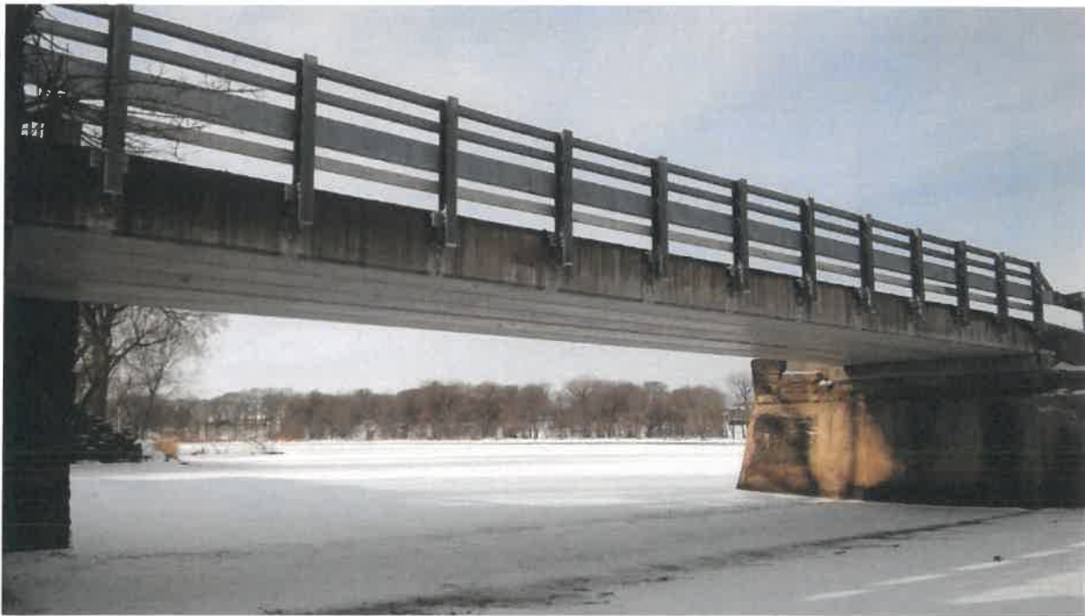
Photo # 8 - Looking south toward west span
