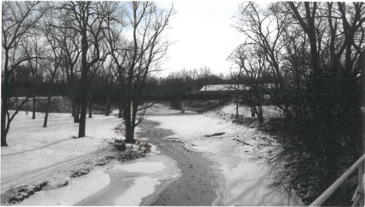
Photo # 2 - Looking upstream from bridge
