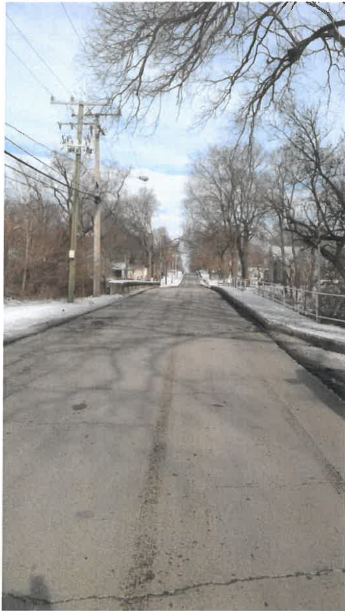
Photo # 1 - Facing north toward bridge
