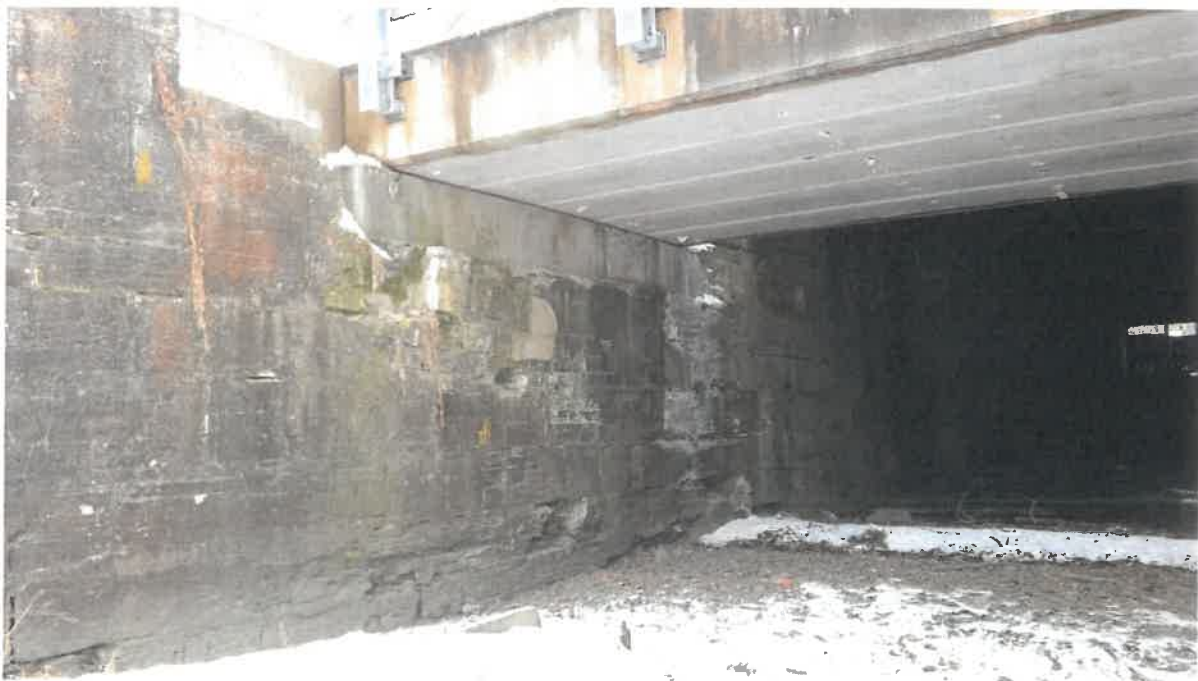
Photo # 5 - Looking southeast toward east abutment
