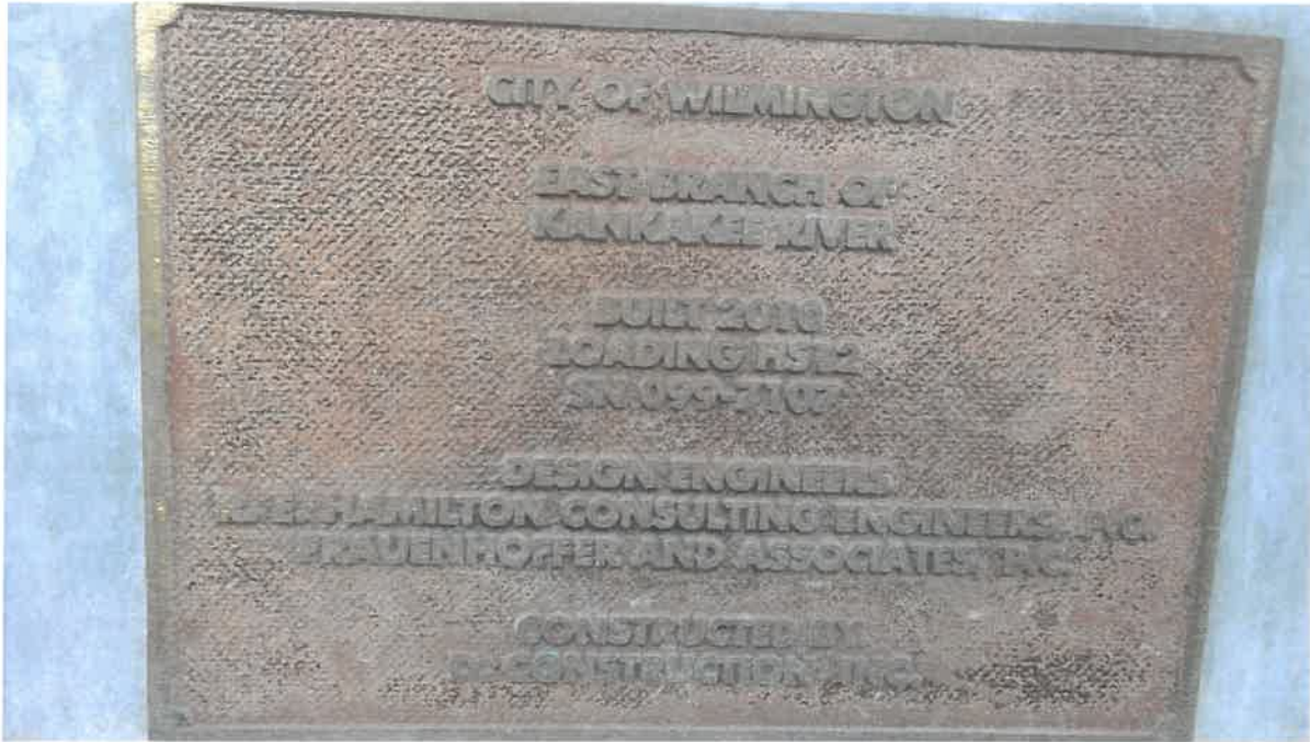
Photo # 13 - Bridge Name Plate
