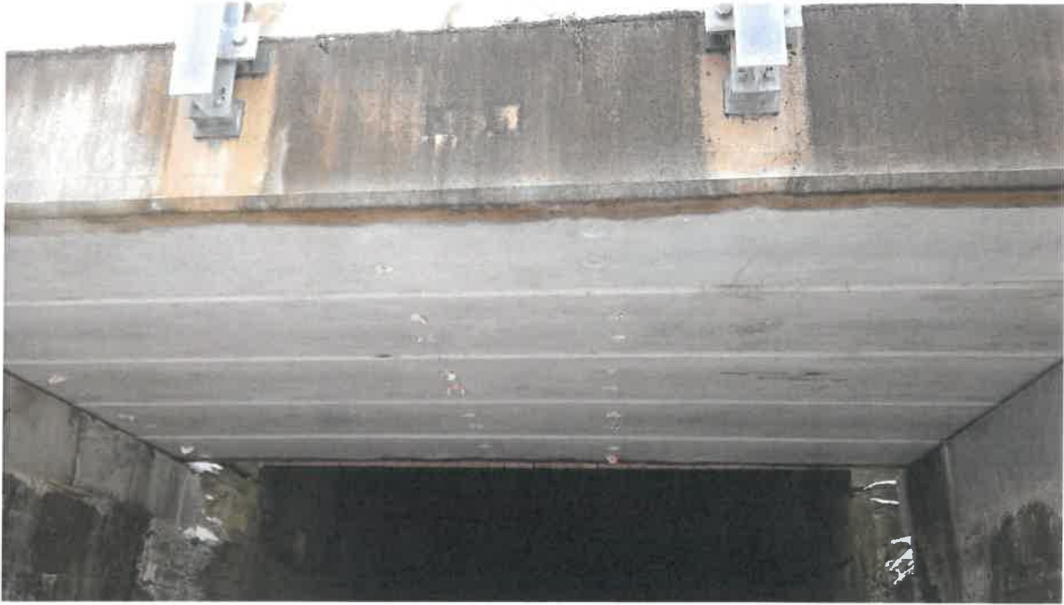
Photo # 7 - Looking south toward east span
