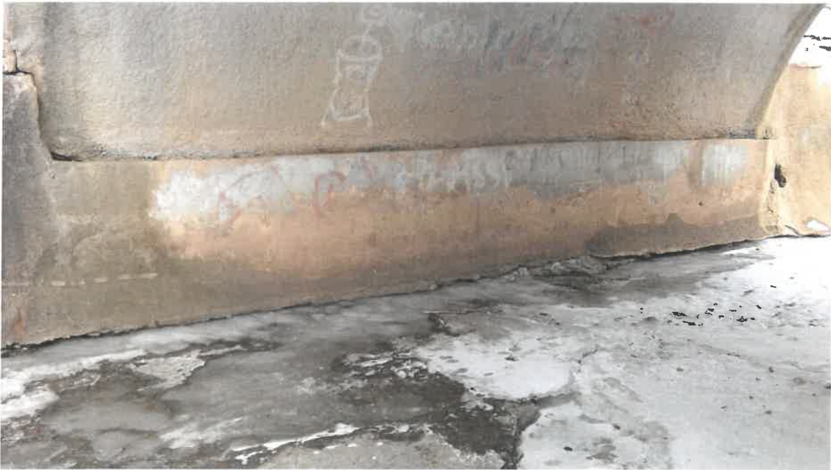
Photo # 8 - Looking northeast toward north abutment
