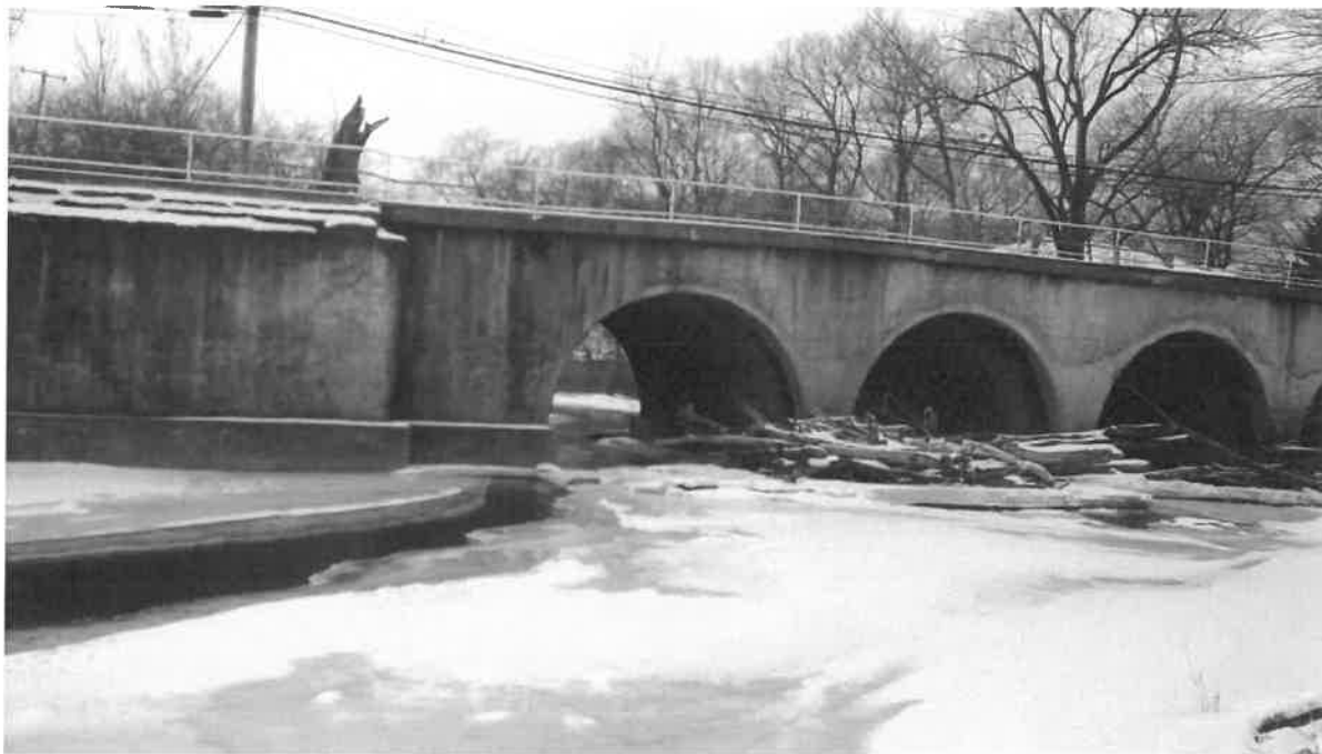
Photo # 9 - Looking downstream toward bridge
