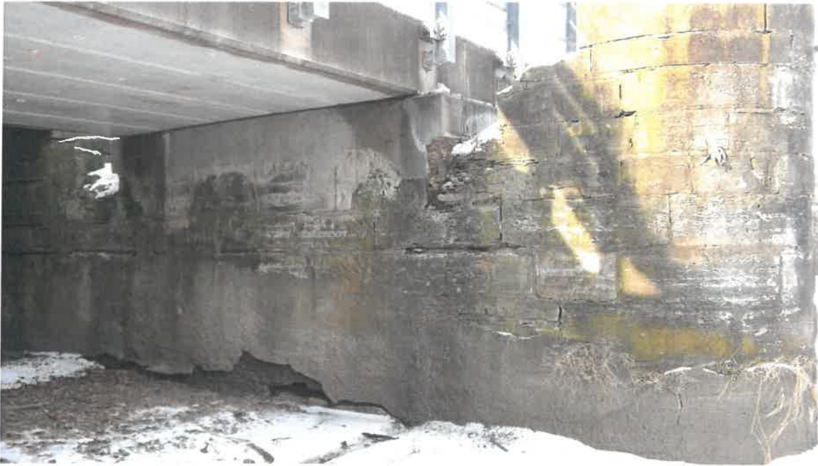
Photo # 4 - Looking southwest toward pier
