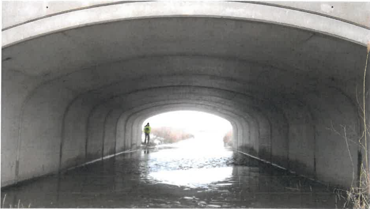
Photo # 6 - Looking upstream thru bridge
