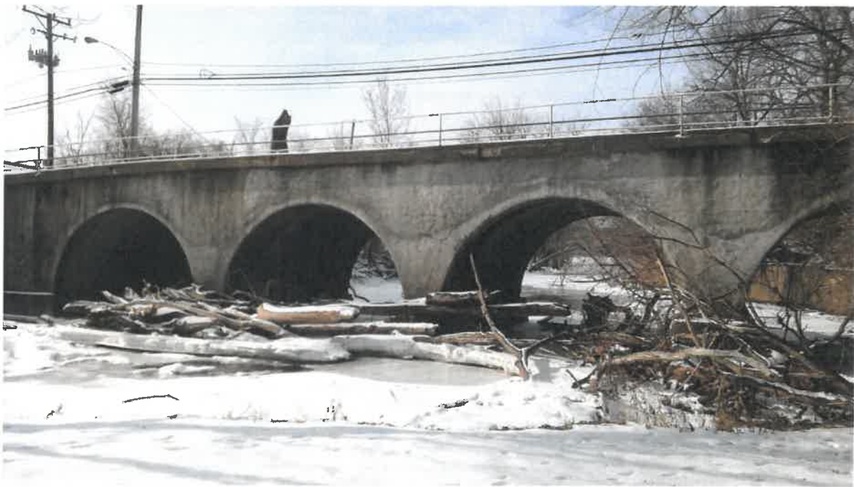
Photo # 5 - Looking downstream toward bridge
