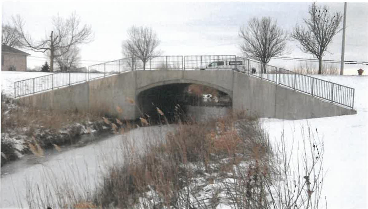
Photo # 7 - Looking downstream toward bridge
