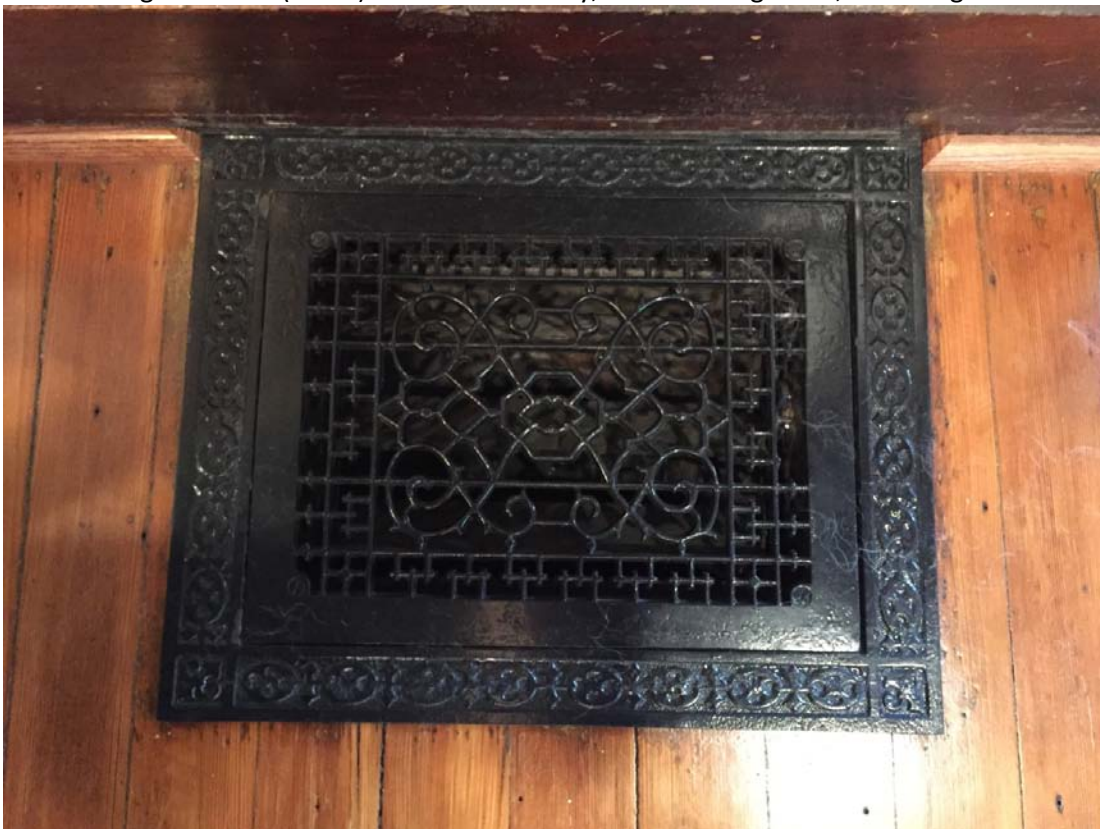
Detail of original floor heating vent grates.
