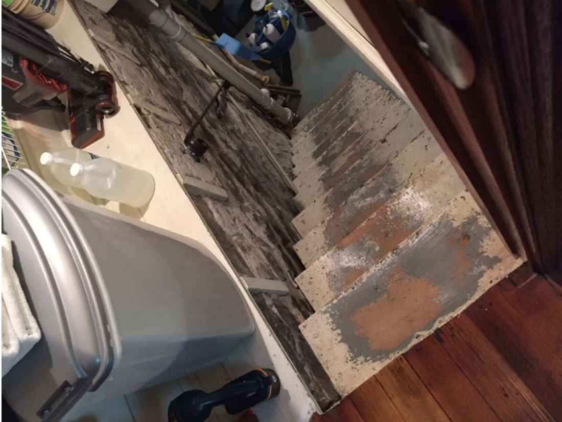
Rear (north) interior steps leading down to basement.
