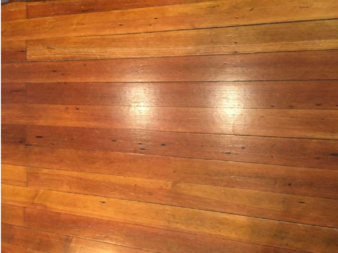
Detail of the original wood floors.
