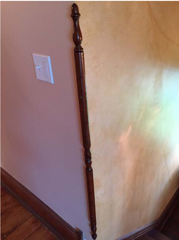
Original wood corner guard in second floor hallway.
