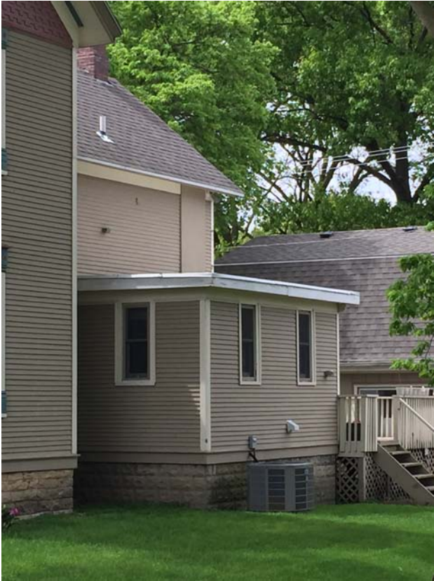
East façade detail of the 1907-1926 addition
