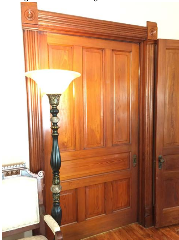
Detail of the large pocket door.
