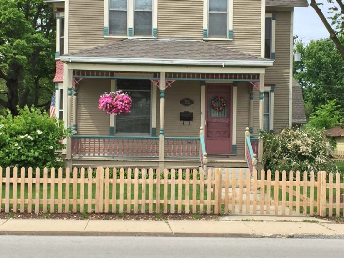
Detail of the porch on the south façade. Note the spindlework porch supports and frieze with brackets.
