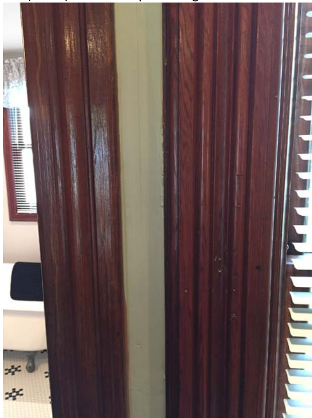
Comparison of the wood door trim – addition on the left and original on the right.
