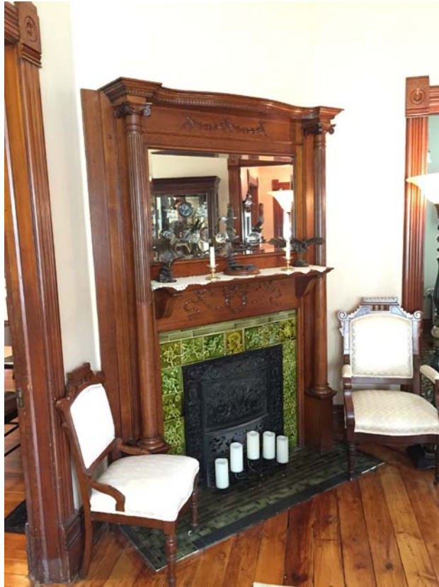
Detail of the original fireplace mantel surround and glazed tile.
