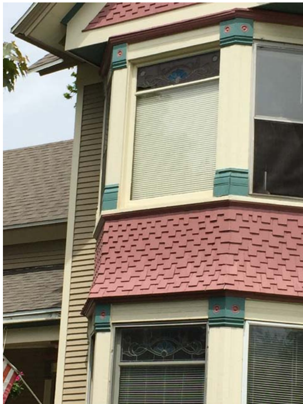
Bay window with art glass and textured shingles; note the gable projects beyond the windows.
