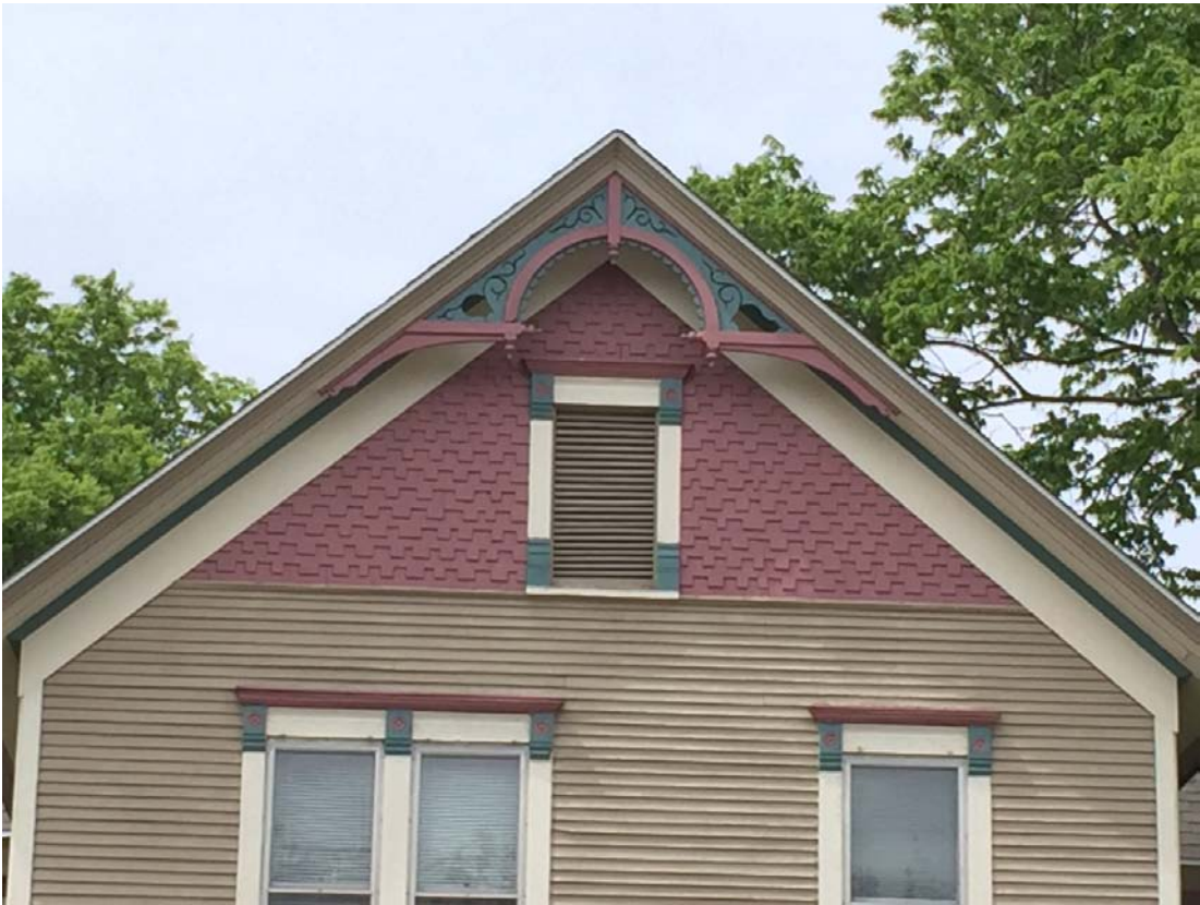
Detail of the siding, textured shingles, and gable bracket
