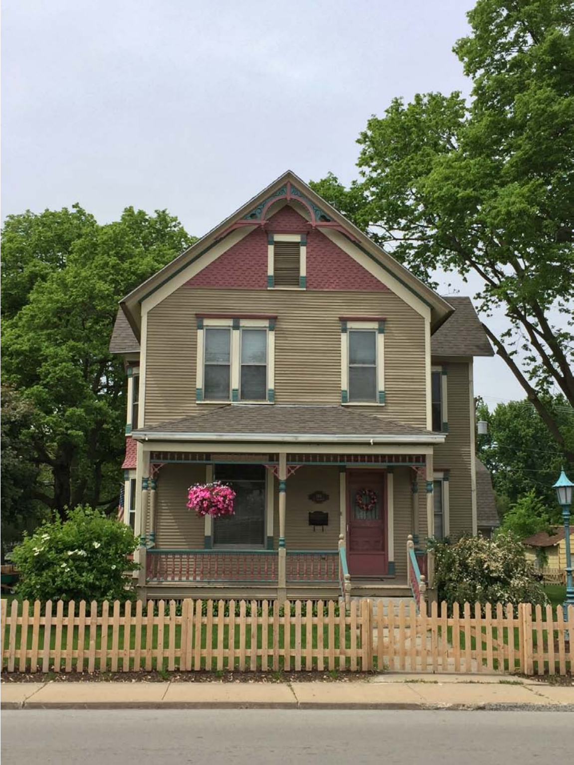
South/Baltimore Street facing façade
