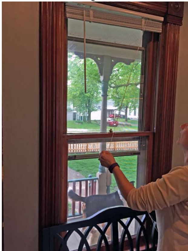
The house retains nearly all its original double hung wooden windows; a few in the rear were replaced.
