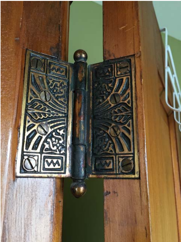
Detail of door hinge, second floor.
